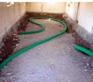
Renewal of the floor: incorporating a radon extract system
