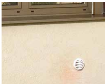
A controlled supply of fresh air creates slightly positive pressure inside rooms/buildings (inside and outside)
