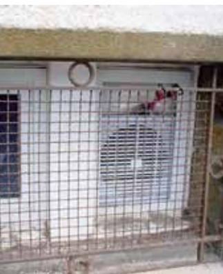
A small fan creates an area of low pressure in the basement or crawl space relative to the inhabited rooms.
