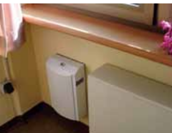
A controlled supply of fresh air creates slightly positive pressure inside rooms/buildings (inside and outside)
