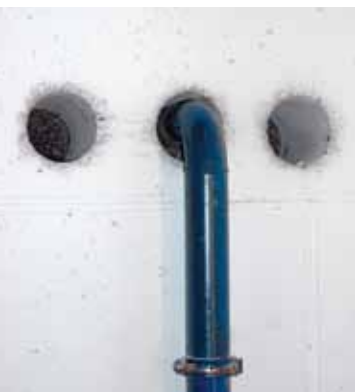
Larger openings and cracks in parts of the building in contact with the soil must be closed.
