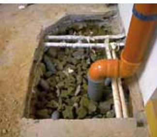
Selective suction (radon suction pit) – digging a pit
