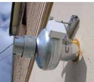
A fan outside the building creates slightly negative pressure under the foundation slab.
