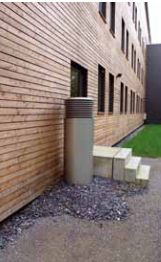
Inlet vent for controlled ventilation of inhabited rooms (at least 80 cm above ground level)
