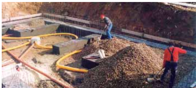
Model on the left: Sub-floor suction, vented through the roof (full-wall pipe with a diameter of at least 15 cm)
