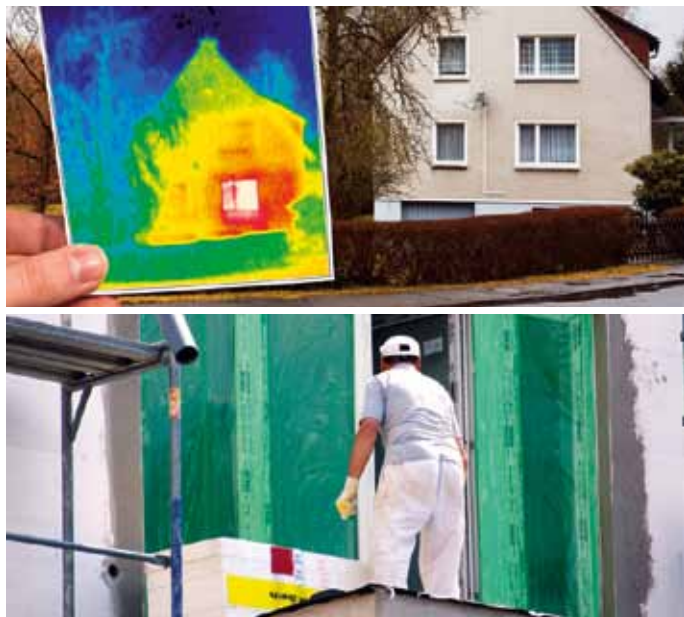
Thermal insulation measures affect the air-tightness of the building envelope.
